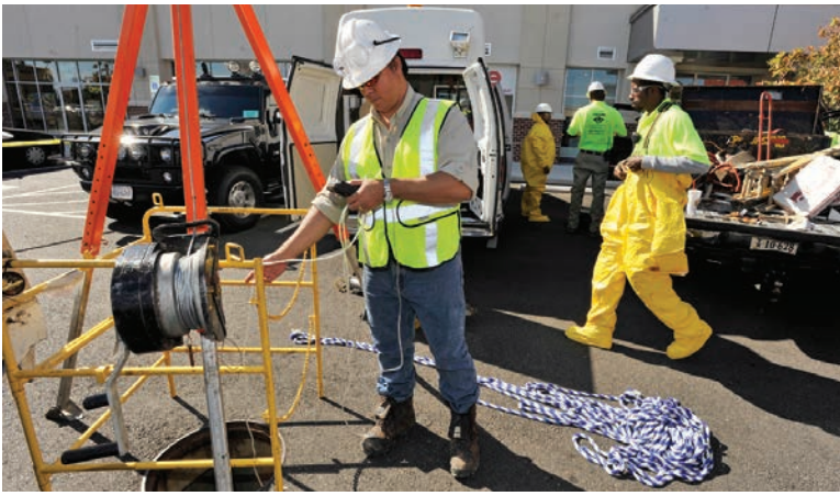
Dave Hawes does an air-quality inspection with the EntryRAE four-gas air monitor unit from RAE Systems before workers go into the confined underground space. At right is Erik Cox as he readies to go underground.
